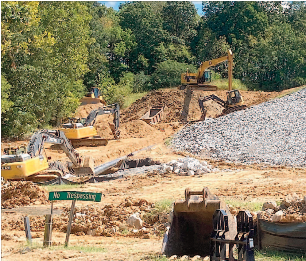
Dry weather has allowed progress to move at a nice pace at Lake George where the levee has been cut on the east end by contractors to facilitate a new syphon pipe. The levee was cut about 15 feet deep for installation. Tim Thomas, Marion’s water crisis consultant, said the contractor was able to install the syphon in segments so that the earthen levee was never completely cut in two, keeping the reservoir from losing additional water. The lake is Marion’s source of raw water. The new syphon will improve the transport of lake water to the nearby plant. A break in the original pipe is believed to have caused some erosion of the dam, leading to the town’s water crisis that became apparent in the spring of 2022. Thomas said Glen Alexander, a Kentucky dam inspector, was here recently to survey the work. Thomas said the progress received good reviews and the inspector was somewhat reassured by quality of interior soil of the dam at the work site. The city, under a governor’s Emergency Order, is being reimbursed by Kentucky Emergency Management for the multi-million-dollar mitigation project at Lake George.
