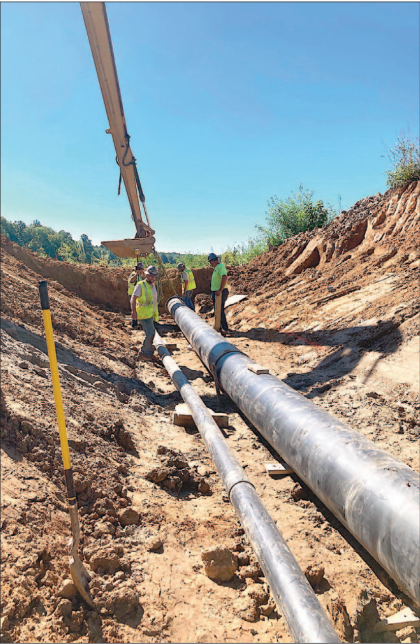
Dry weather has allowed progress to move at a nice pace at Lake George where the levee has been cut on the east end by contractors to facilitate a new syphon pipe. The levee was cut about 15 feet deep for installation. Tim Thomas, Marion’s water crisis consultant, said the contractor was able to install the syphon in segments so that the earthen levee was never completely cut in two, keeping the reservoir from losing additional water. The lake is Marion’s source of raw water. The new syphon will improve the transport of lake water to the nearby plant. A break in the original pipe is believed to have caused some erosion of the dam, leading to the town’s water crisis that became apparent in the spring of 2022. Thomas said Glen Alexander, a Kentucky dam inspector, was here recently to survey the work. Thomas said the progress received good reviews and the inspector was somewhat reassured by quality of interior soil of the dam at the work site. The city, under a governor’s Emergency Order, is being reimbursed by Kentucky Emergency Management for the multi-million-dollar mitigation project at Lake George.
